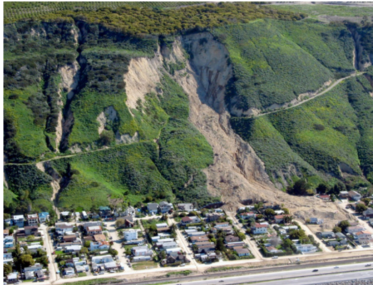
Figure 1.1 The 2005 La Conchita Landslide, Ventura County, California, killed 10 people and destroyed 36 homes.
